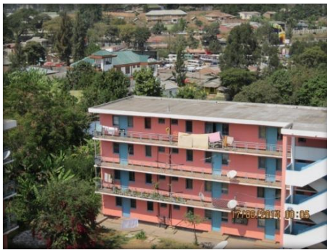
Figure 3. Mbeya City Morphology- Around Bus Terminal Area Highlighting Building heights and Landscape.
